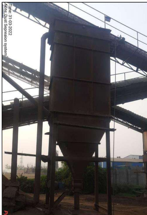
Dust Suppression System
